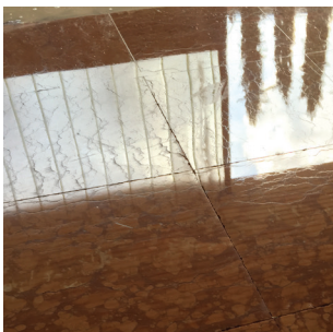
Example of usage on marble surfaces, from roughing with diamond-coated metal grinding disc to high gloss polishing with TMB SHINEPAD disc
